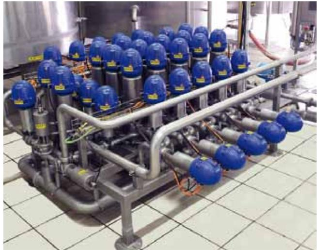
Moloko Dairy cream valve cluster with Alfa Laval Unique SSV, Unique Mixproof and LKB valves and ThinkTop valve sensing and control units.
